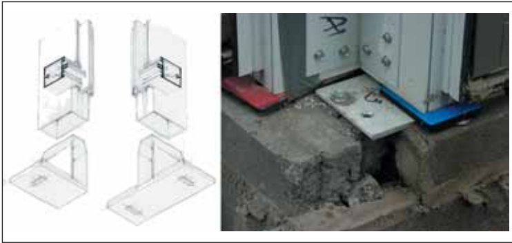
Figure 8. Examples of transom discontinuity.
